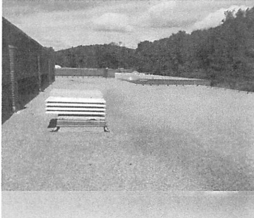
Photo #1: Overview of the West side of the School, Section E
